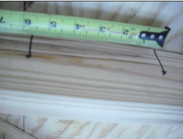
Roof deck attachment
