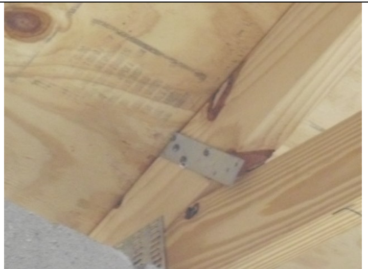
Roof to wall attachment
