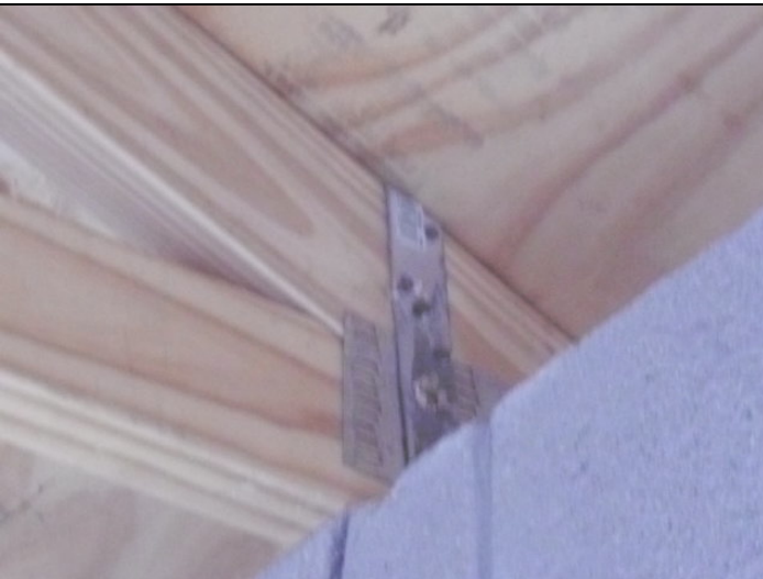
Roof to wall attachment
