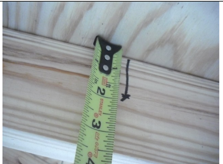
Roof deck attachment
